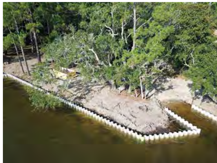
A total of 222-feet of seawall is being replaced as part of the Kellogg Park renovation project. Work on the park, which is located on the southern portion of the Choctawhatchee Bay near the Clyde B. Wells Bridge, is about 90 percent completed.
