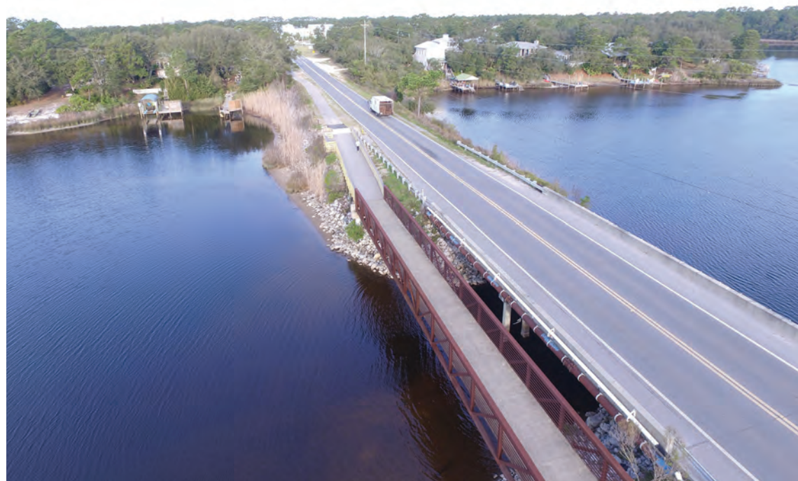
As part of the Walton County TDC's capital improvement project, wooden pedestrian bridges at Eastern Lake, pictured above, Draper Lake and Deer Lake were renovated, as Deer Lake was replaced with new metal spans and the wooden sections of Eastern Lake and Draper Lake were replaced.
